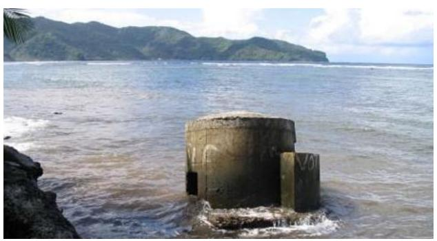
**Figure S.MH.14.5.** World War II pillbox defensive structures are located along the shorelines of Tutuila, where they are slowly being impacted by coastal erosion. Photo: Hans Van Tilburg/NOAA
