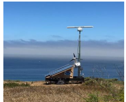
A shore-based radar system at Santa Cruz Island. Photo: NOAA.
