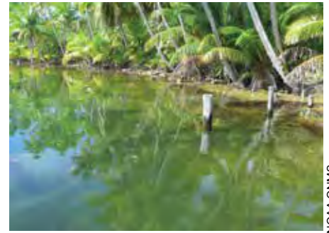
Figure 91: Three wooden pilings extending out from the southern shore of the lagoon, one submerged.
