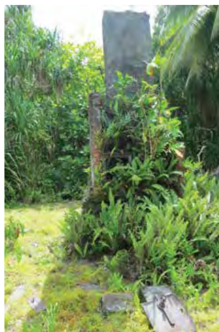
Figure 201: Oven within cookhouse stone chimney.
