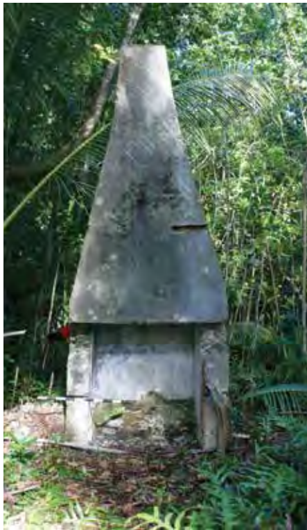
Figure 130: Chimney site near cut beach rock path. Chimney faces east.
