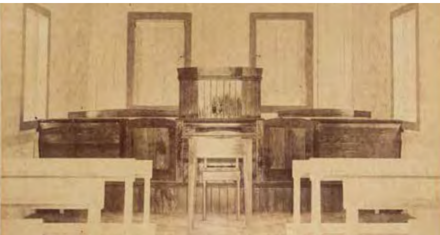
Figure 180: Interior of Taulaga church showing the appearance of the altar area in 1889.
