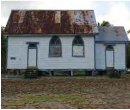
Figure 174: North side of church at Taulaga 2013.
