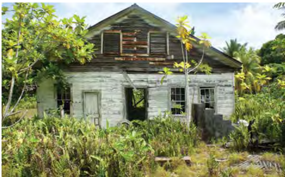
Figure 147: Back of Jennings residence and concrete steps.
