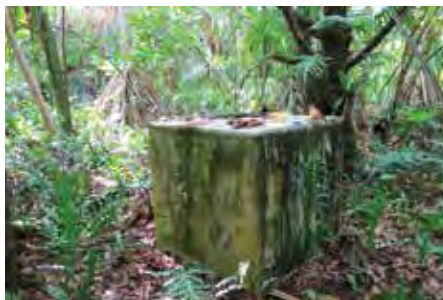
Figure 195: Tank #2 (peninsula road).
