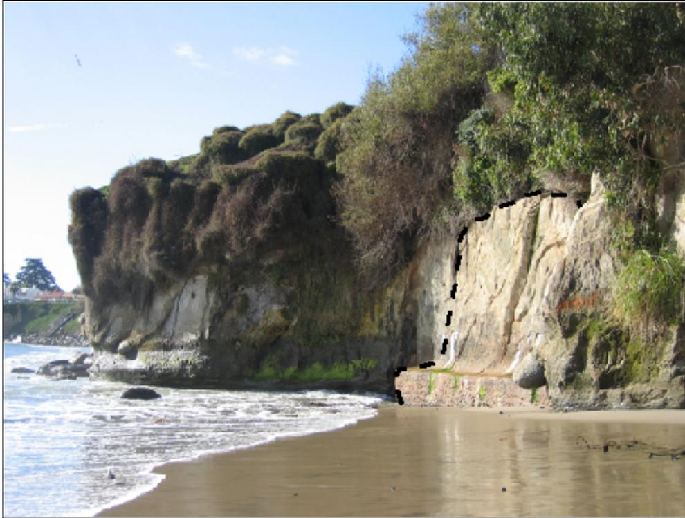
Figure 4: Photograph of cliff stabilization built to fill a seacave at Cowell's Beach in Santa Cruz. The 2004 gunitite wall, outlined by the black dashed line, mimics the shape and color of the natural cliff.
