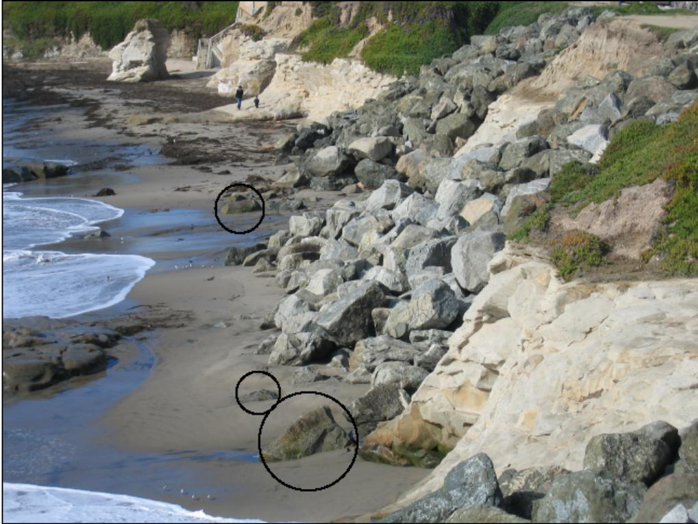
Figure 9: Riprap boulders commonly settle into deep sandy beaches or get buried, as seen here near the intersection of Westcliff Drive and David Street in Santa Cruz, California.
