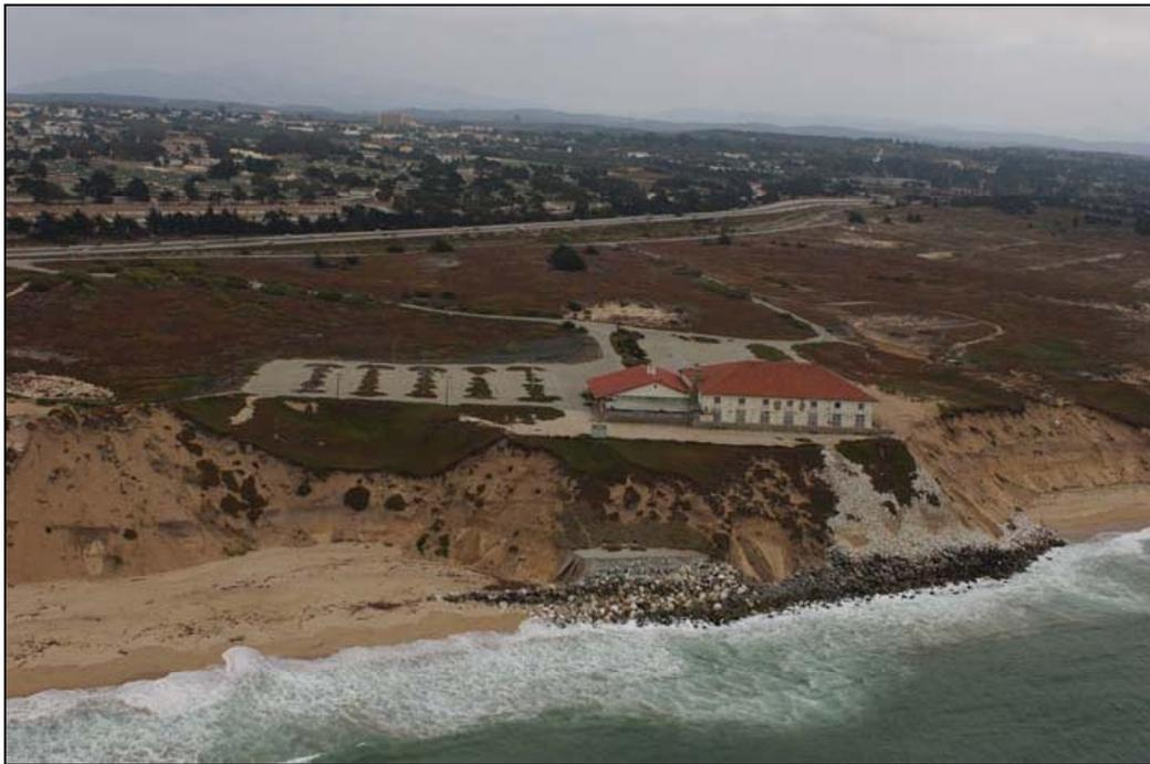
Figure 1a: Oblique aerial photograph of Stillwell Hall in 2002 in Marina, CA. Coastal protection structures placed at the base of the aged building were neither effective nor efficient enough keep up with intense coastal erosion of adjacent bluffs. Photograph copyright © 2002 Kenneth & Gabrielle Adelman (<http://www.californiacoastline.org/>).
