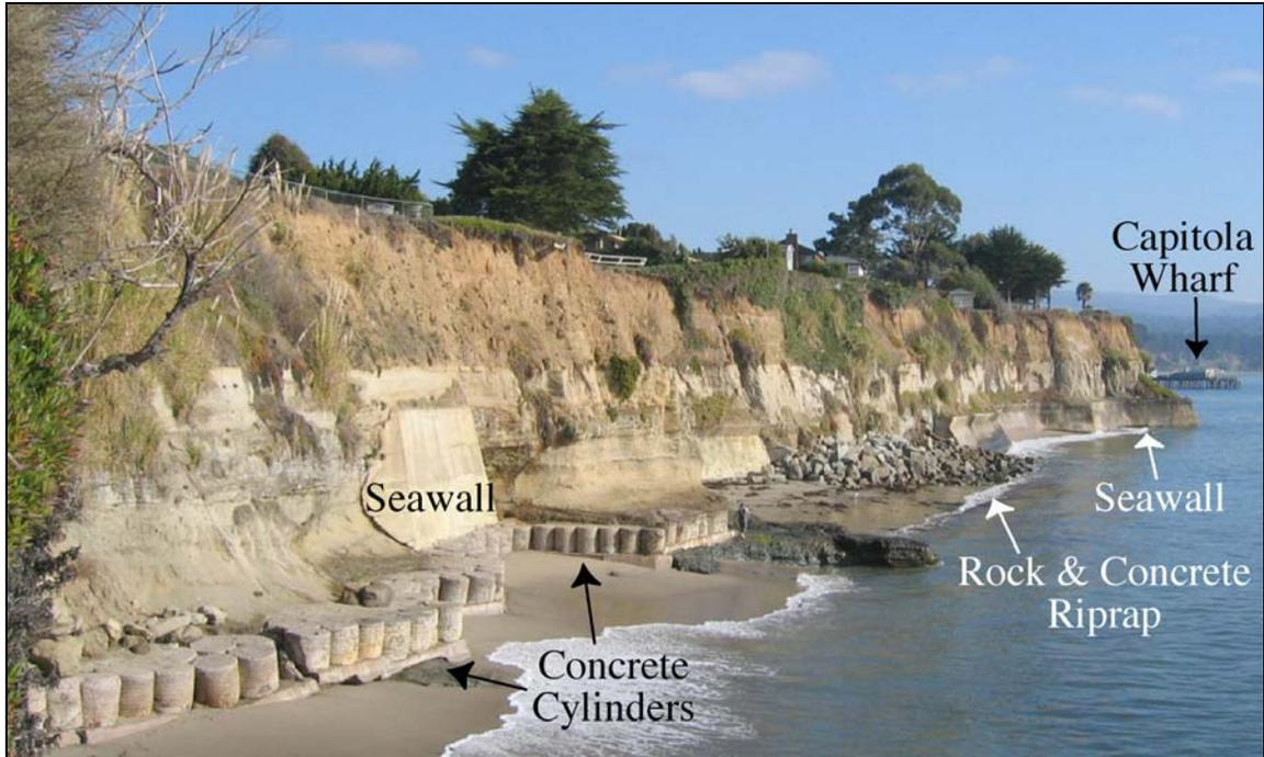
Figure 3: An unplanned assemblage of coastal armoring at Opal Cliffs in Capitola, California can have a visual impact on the beach user.
