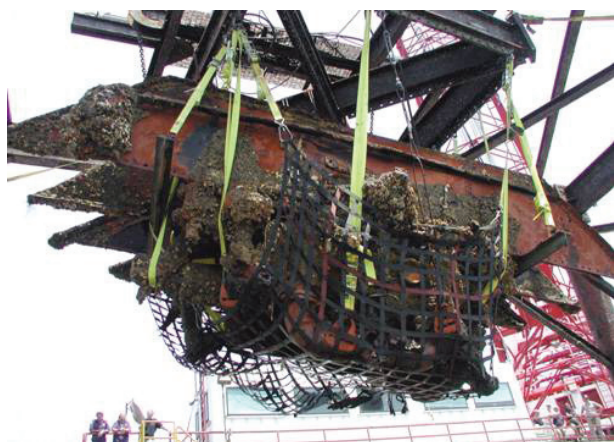
Recovery of the engine will permit researchers a unique opportunity to study builder John Ericsson's innovative vibrating side-lever engine.
