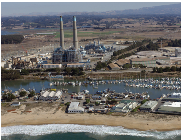
Figure 21. The power plant in Moss Landing contains a desalination plant that produces fresh water for use in the power production process.
