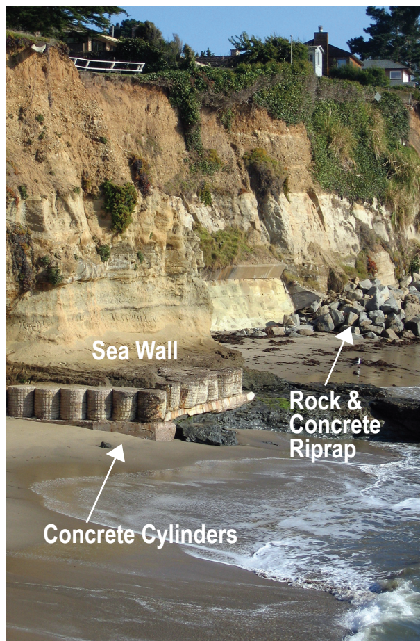
Figure 81. An unplanned assemblage of coastal armoring structures at Opal Cliffs near the city of Capitola (on the north side of Monterey Bay).
