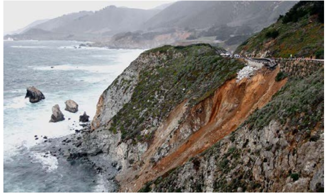
Landslide in Big Sur, with slide debris entering the MBNMS.
