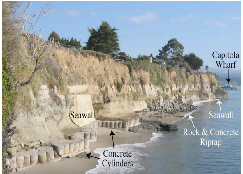
Examples of coastal armoring structures near the city of Capitola (on the north side of Monterey Bay). Image credit: MBNMS
