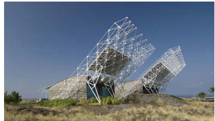
NELHA Gateway Energy Center in Kona / Photo Source: Ferraro Choi and Associates
