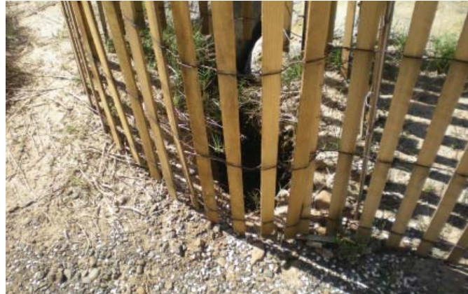
Existing shoreline erosion / Photo: FCA
