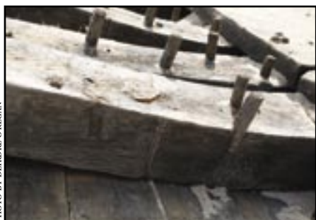
Trunnels (treenails) and trunnel wedges protrude from the massive frames.
